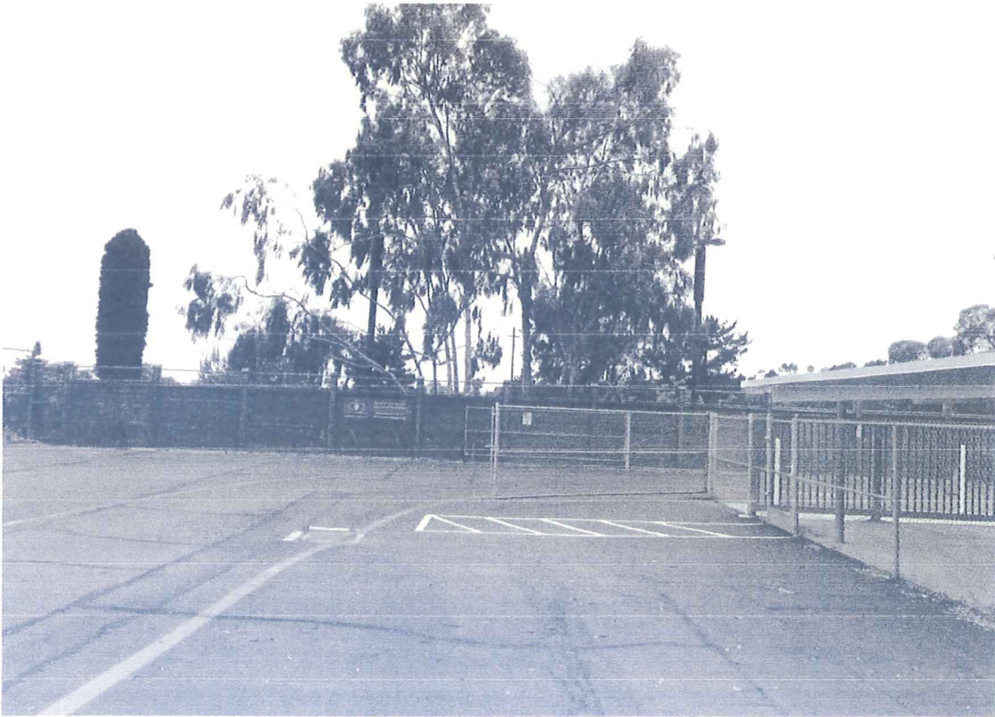
3. View of East Elevation of site.
