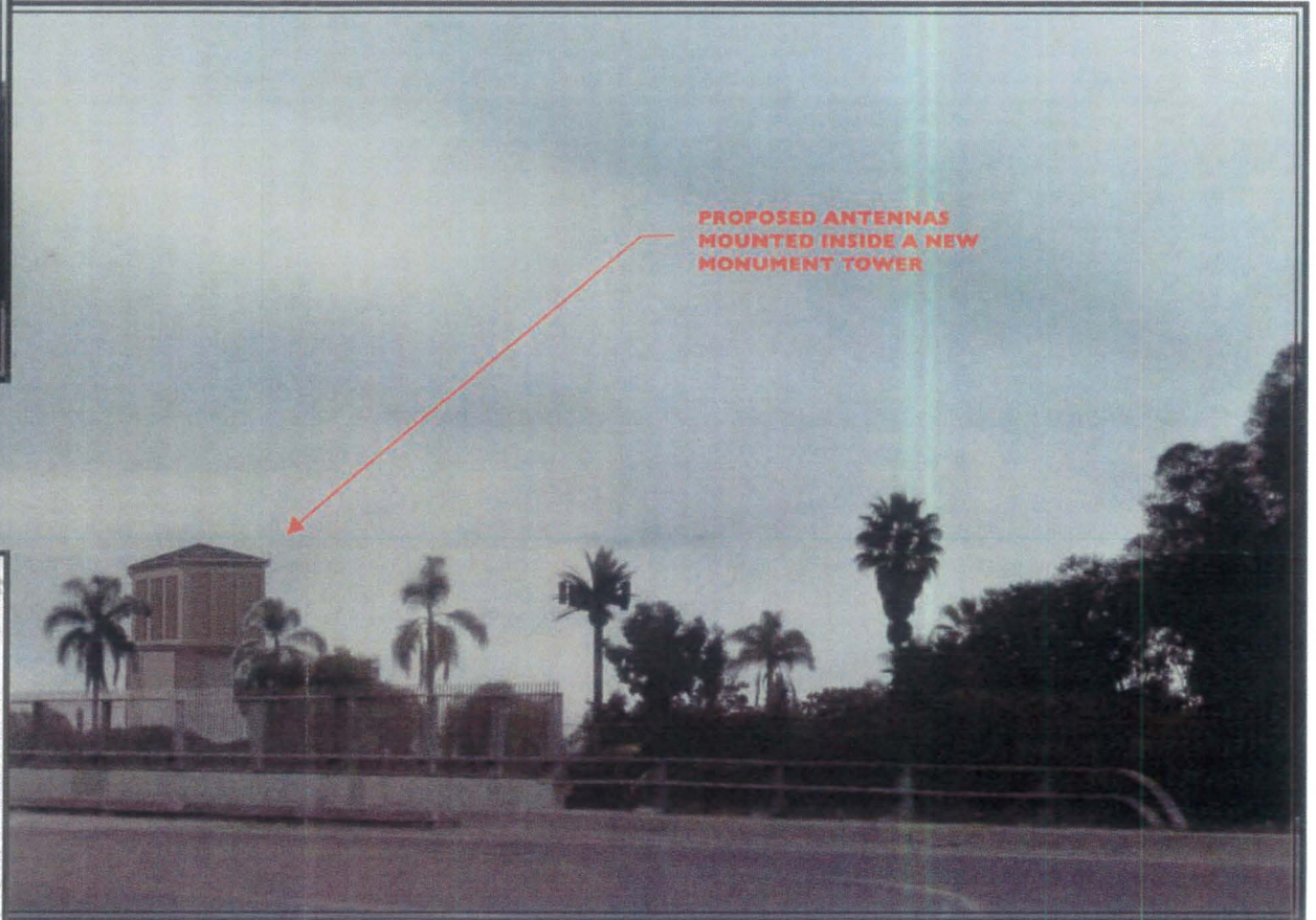
SITE AFTER INSTALLATION
