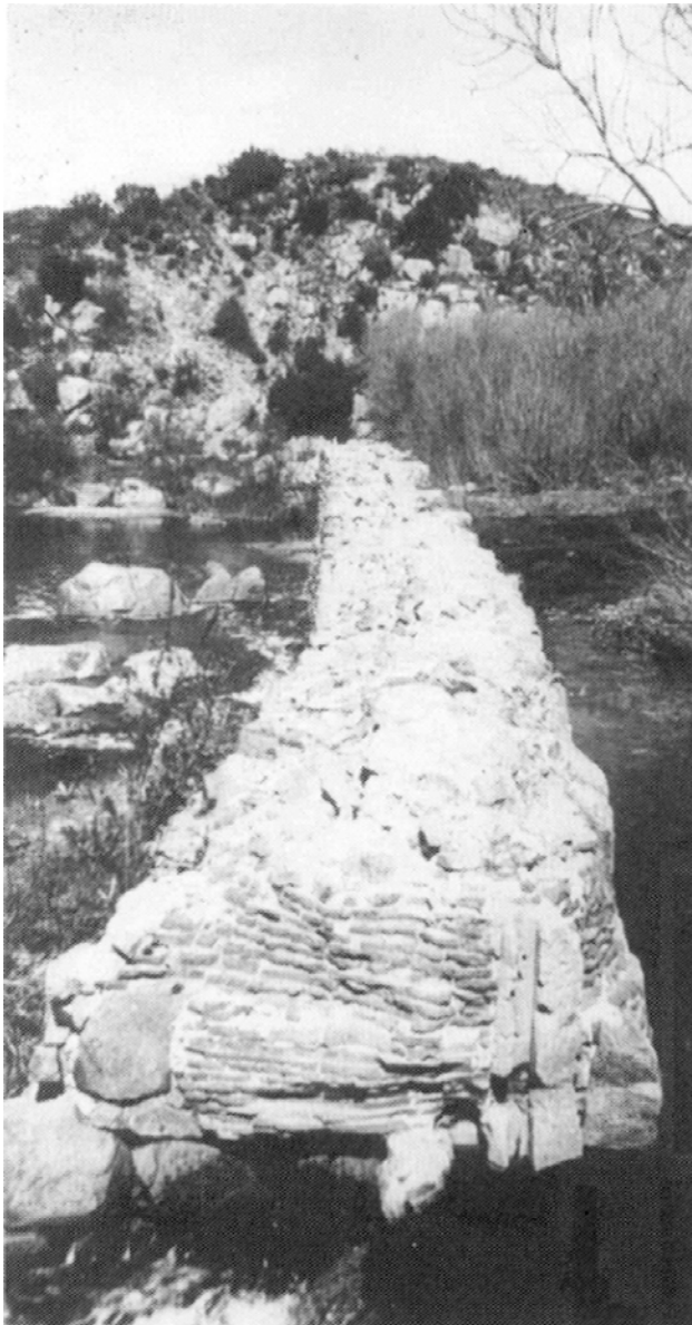
Remaining structure of the old mission dam built in the 1700s to provide water for irrigation
