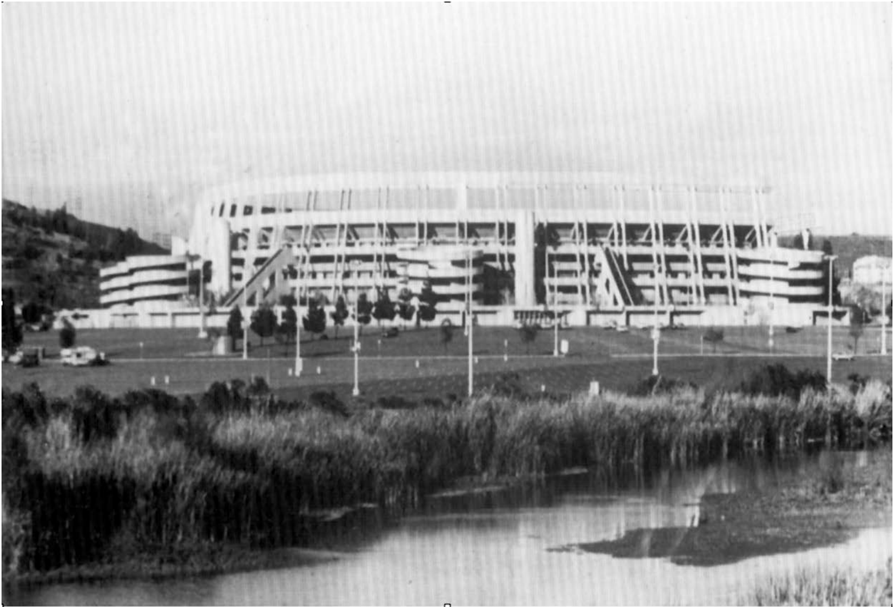
San Diego Jack Murphy Stadium as seen from the river channel
