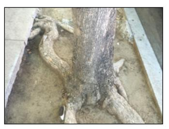
Soil compaction causing surface roots and sidewalk damage
