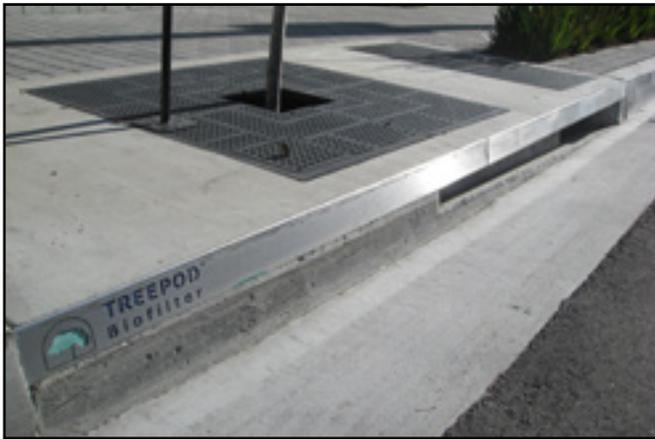
TreePod Biofilter Installation
