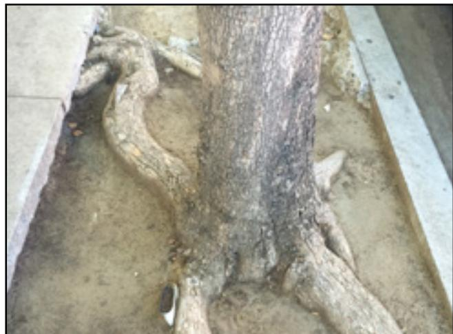
Soil compaction causing surface roots and sidewalk damage
