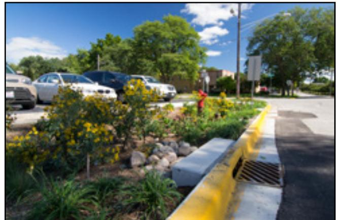
Filtering runoff with plant material
