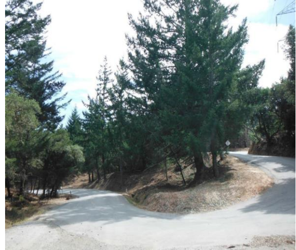
Figure 4. San Mateo County – Mechanized – After
