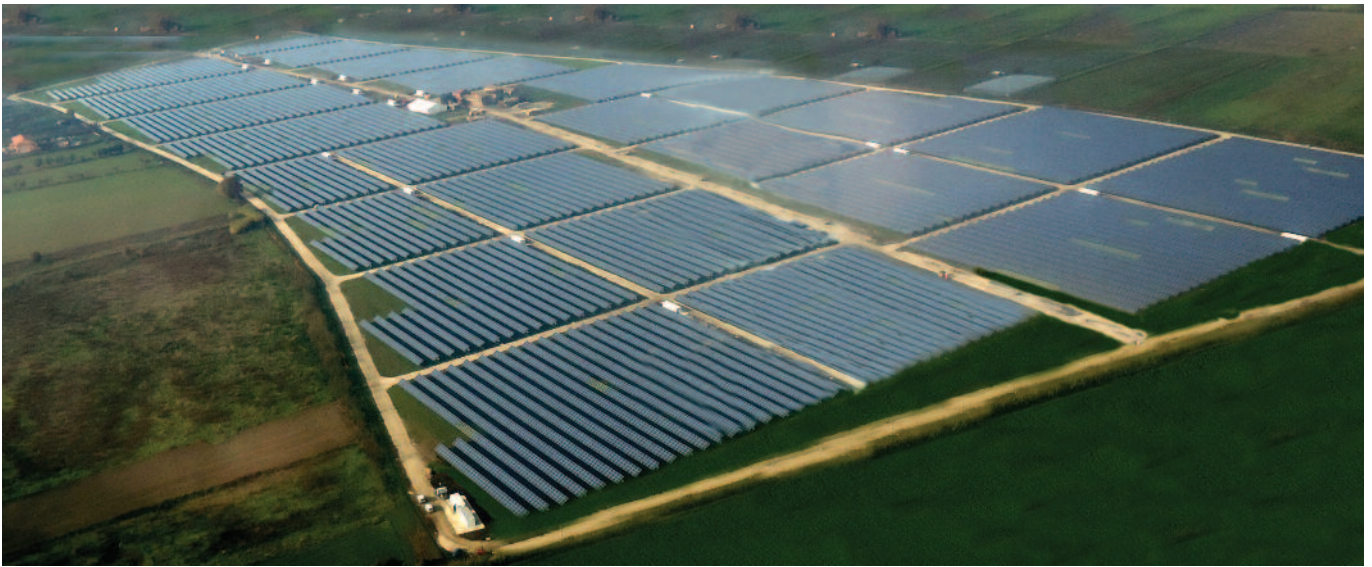
Solar energy park in Campania, Italy
