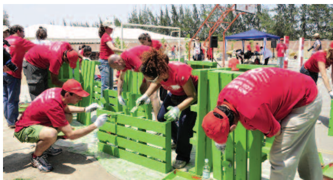
Volunteers helping to build homes in Chile
