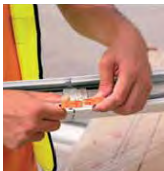
8th and 9th wire: tool-less through-wiring via click.
