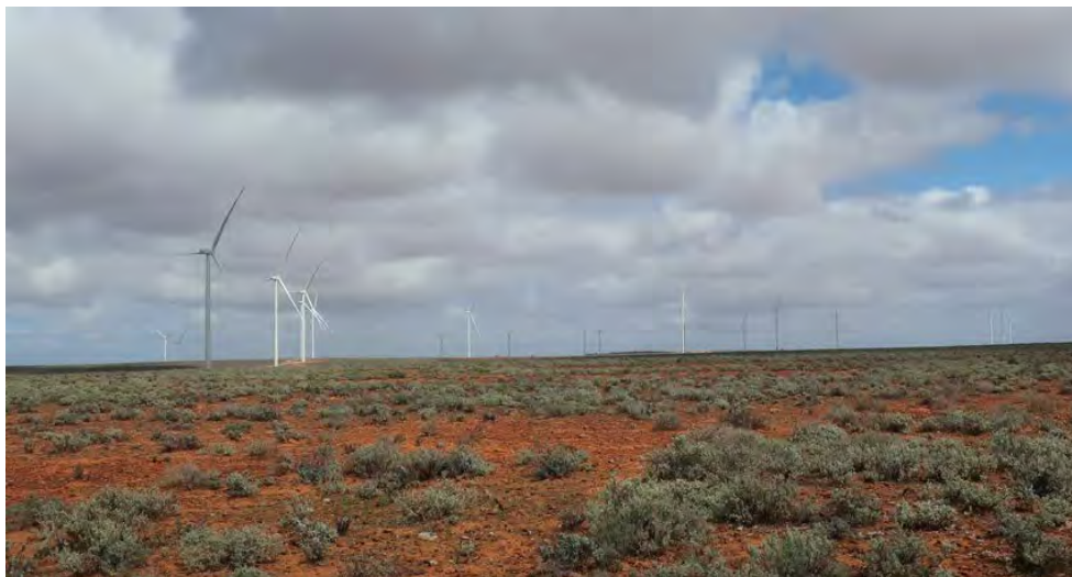
Constructed Turbines – Stage 1: Lincoln Gap Windfarm
