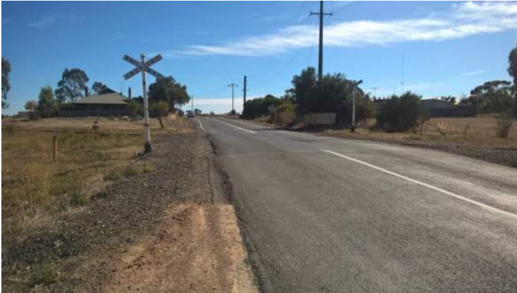
Photo 7.15 Barrier Highway – Min-Man Road junction looking north
