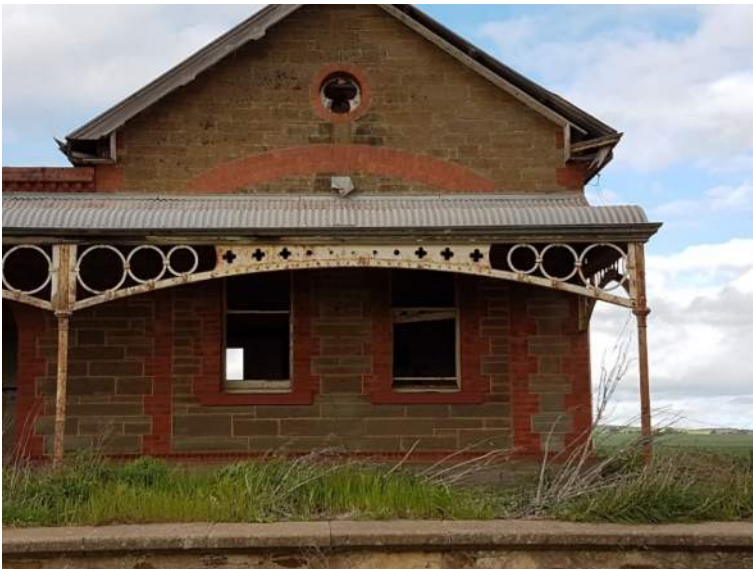
Photo 7.9 Merildin Railway Station (renamed from 'Mintaro' in 1918) - located one kilometre away from the project site boundary
