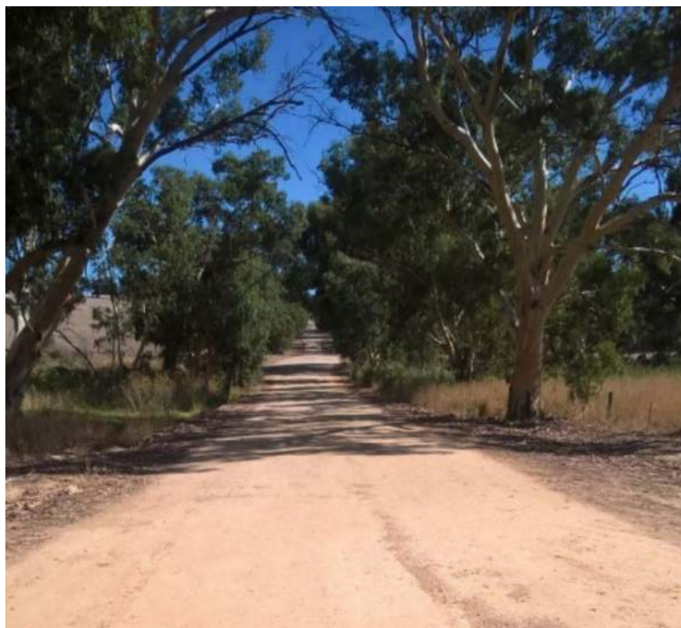
Photo 7.13 Hare Road looking north towards the uphill grade
