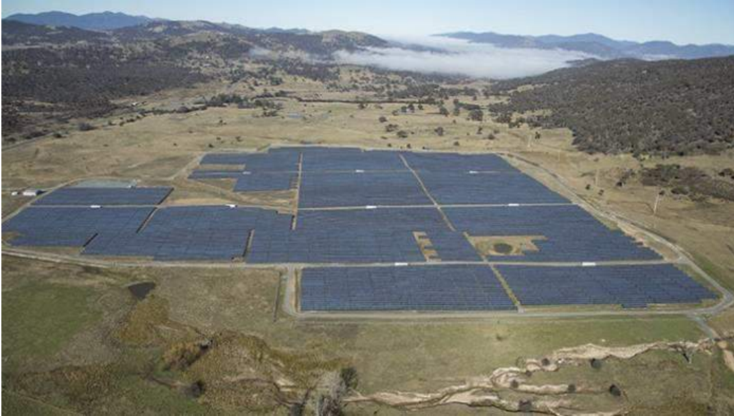
Solar: Royalla Solar Farm (ACT). Photo: royallasolarfarm.com.au
