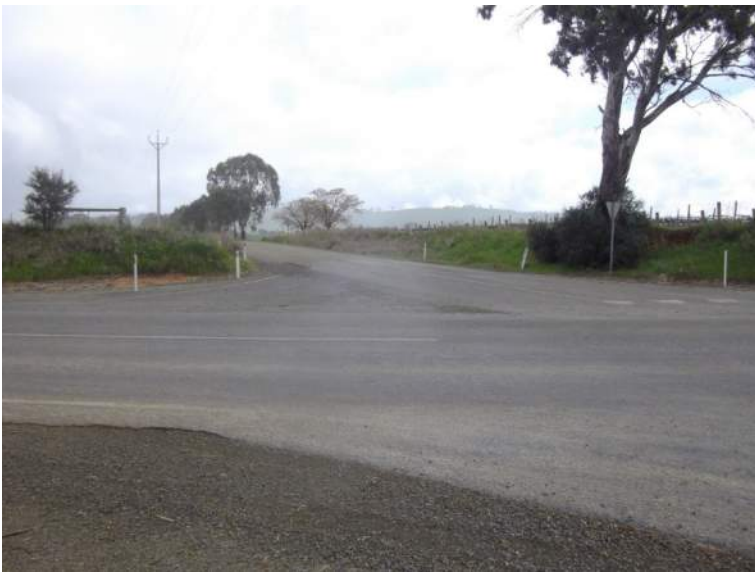
Photo 7.14 Intersection of Copper Ore Road and Mintaro – Merildin Road
