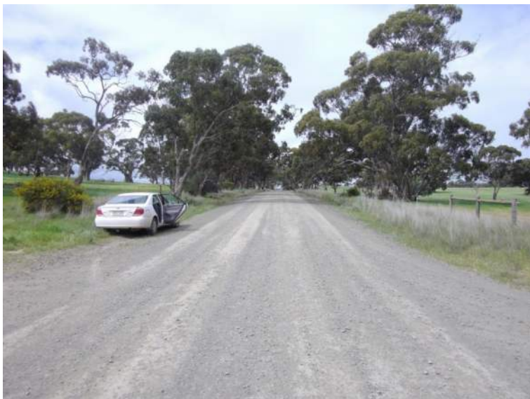
Photo 7.10 Mintaro – Merildin Road (looking west from intersection with Wookie Creek Road)
