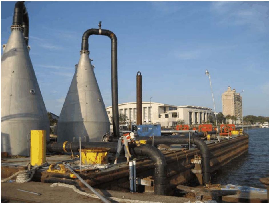
Figure 4. Speece Cones set up as Demonstration Project on the Savannah River
