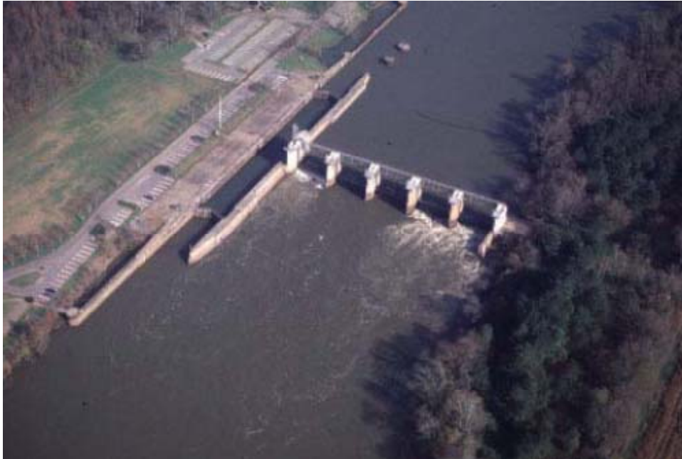
Figure 22. New Savannah Bluff Lock and Dam
