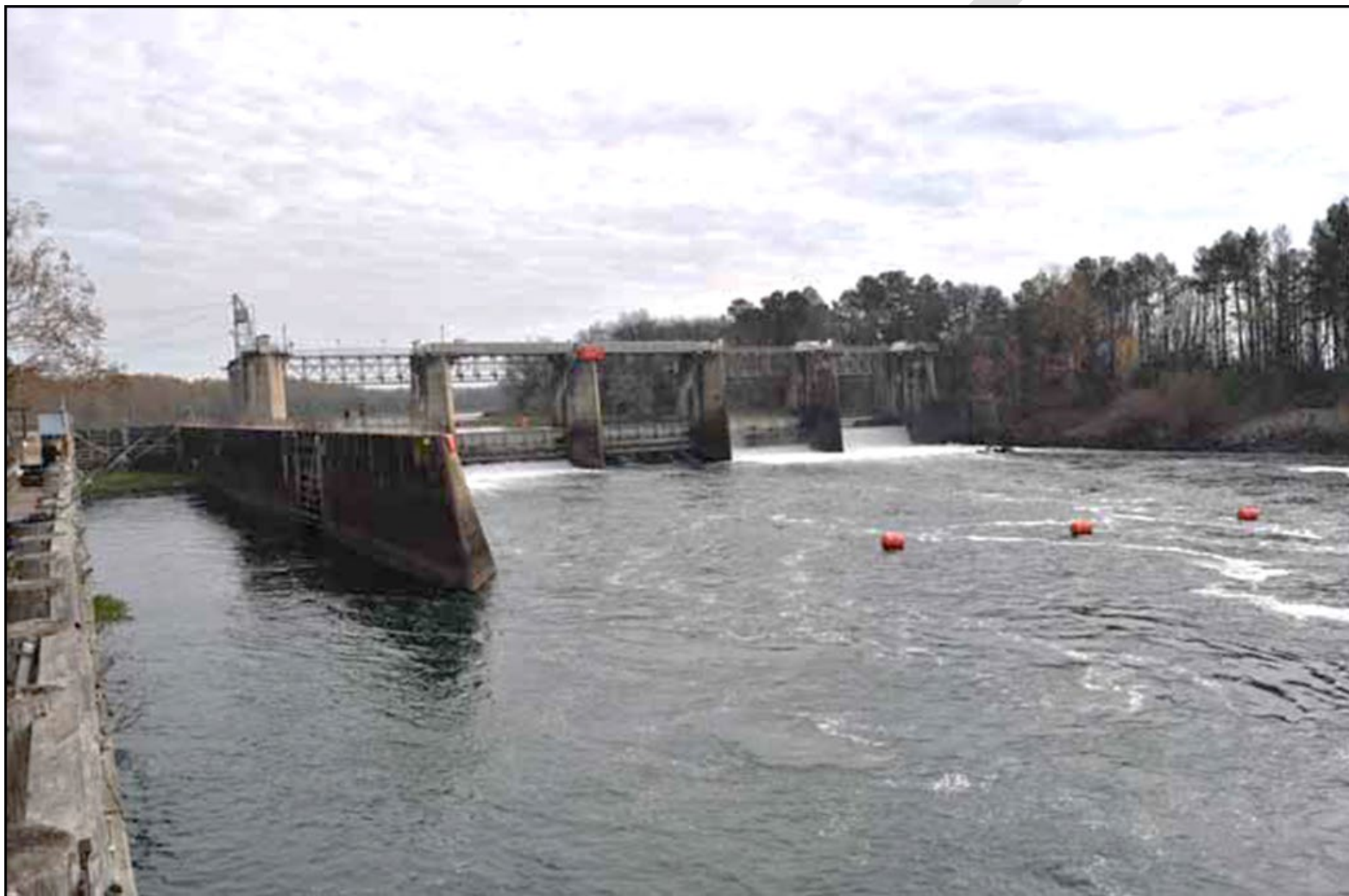
Figure 4. Photograph of downstream side of New Savannah Bluff Lock and Dam
