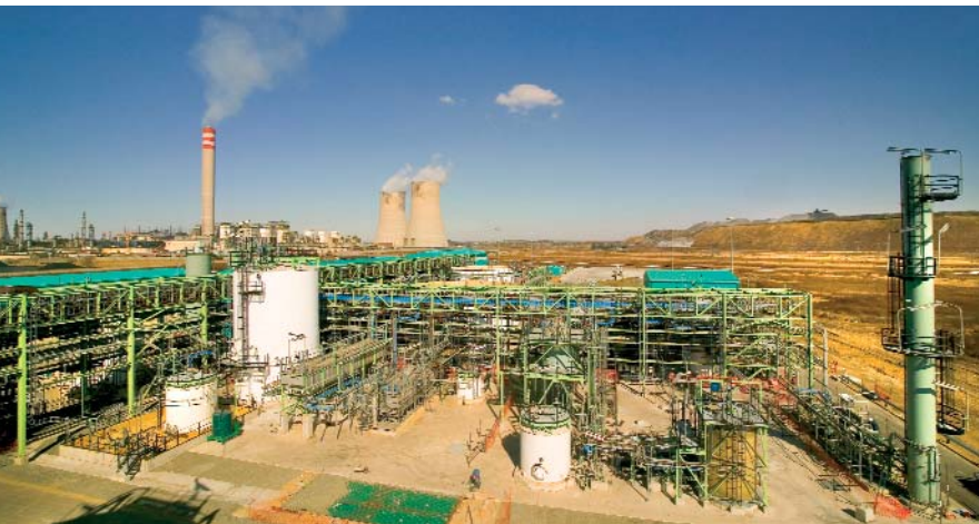
Sasol is undertaking several major investments to improve its waste-management facilities and environmental performance.
