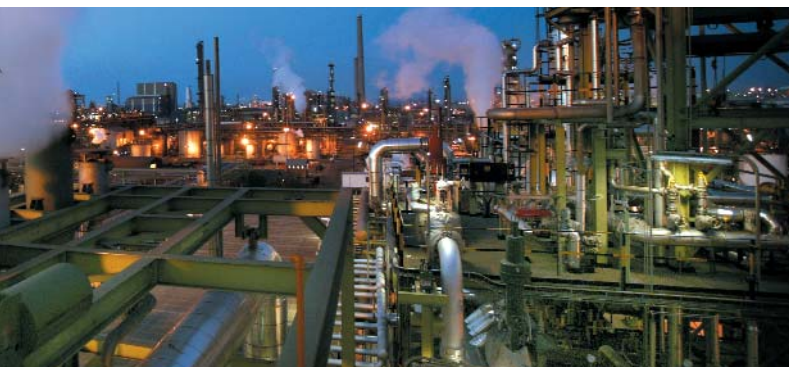
Two autothermal reformers at Sasolburg reform natural gas into synthesis gas.
