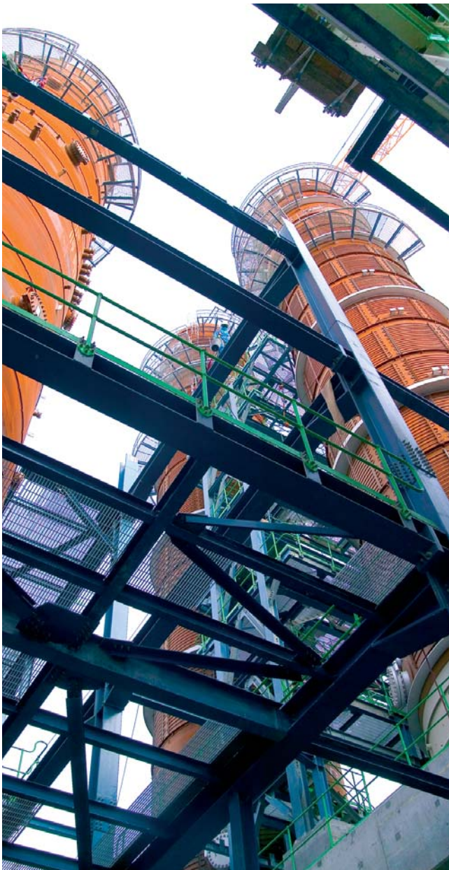
The Oryx GTL plant is one of the group's major new investments being executed with expert support from Sasol Financing.
