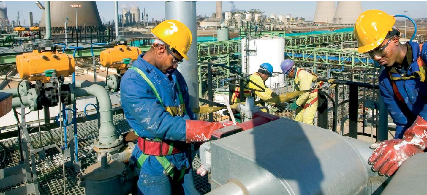
A new Sasol waste-recycling facility under development at Secunda in South Africa.
