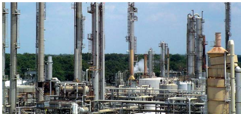
Merisol cresylics plant at Greens Bayou in Houston, USA.
