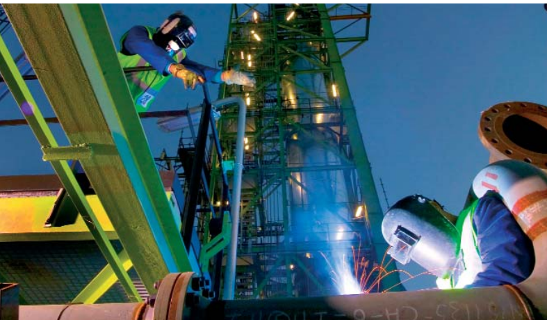
A view of the third 1-octene plant at Secunda, South Africa.
