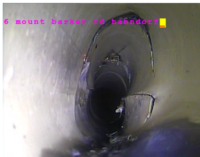
Large tree roots causing wastewater pipes to crack in search of water. Left photo: clay pipe. Right photo: PVC pipe.
