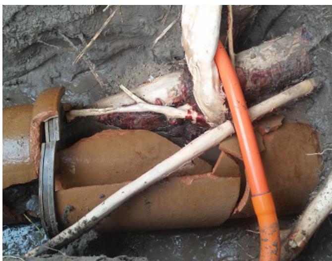
Large tree roots causing wastewater pipes to crack in search of water. Left photo: clay pipe. Right photo: PVC pipe.
