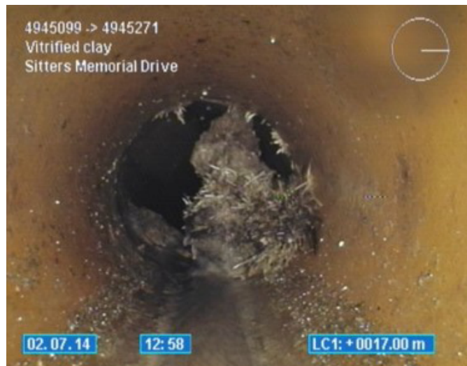
Closed Circuit Camera Television image inside a wastewater pipe as fine hair tree roots penetrate pipe joints in search of water.
