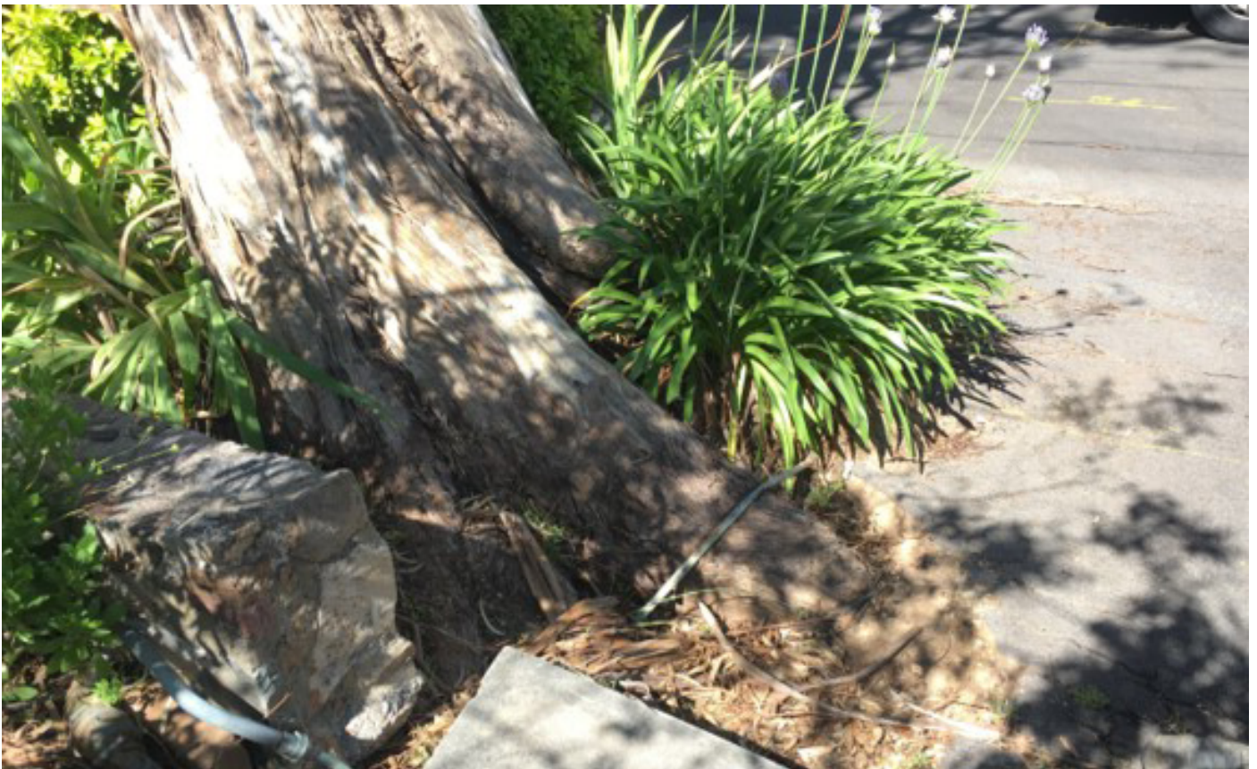
Tree root lifting a customer water connection.
