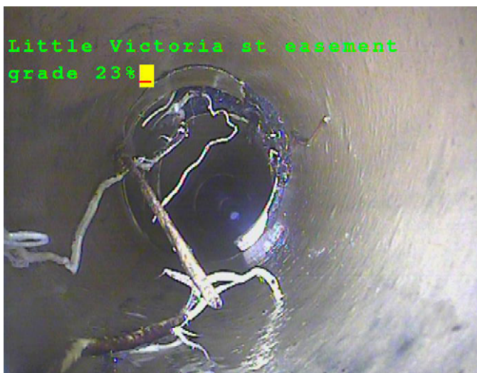
Closed Circuit Camera Television image inside a wastewater pipe as fine hair tree roots penetrate pipe joints in search of water.
