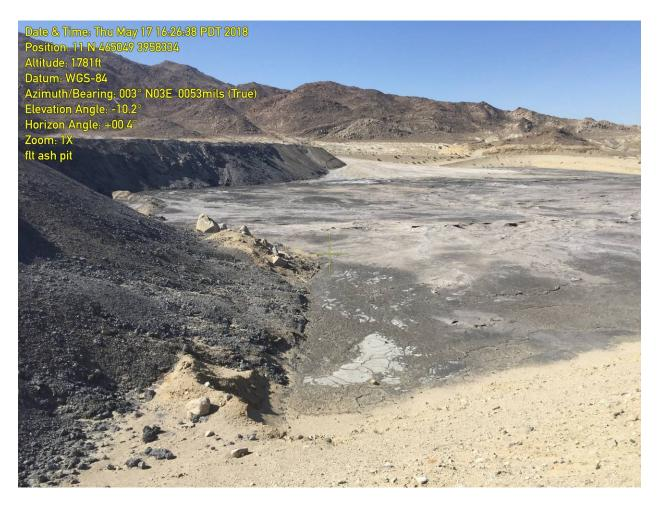
Photograph 2. PVL Lime Plant Project – view of open Cell #5 showing disposed ash
