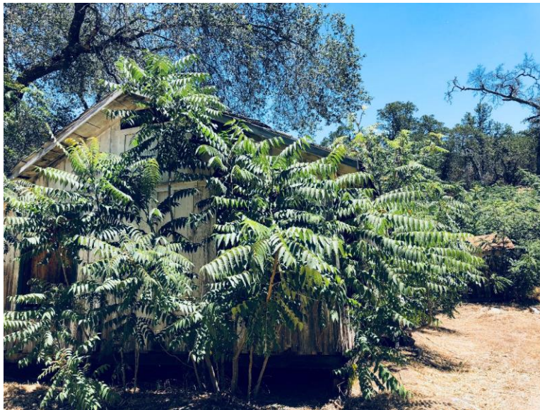
Photo I-8 Tree of heaven ( Ailanthus altissima ) along the Kaweah No. 3 Powerhouse to Three Rivers Substation Transmission Line.
