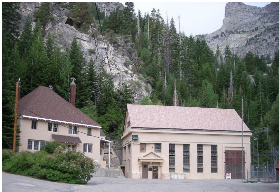
Photo 4.5-3. Poole Powerhouse and Residence
