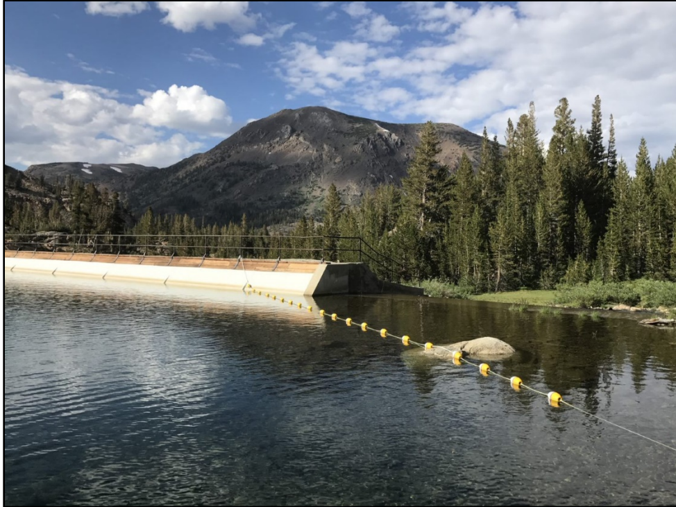
Photo 5.10-3. Tioga Dam and Spillway
