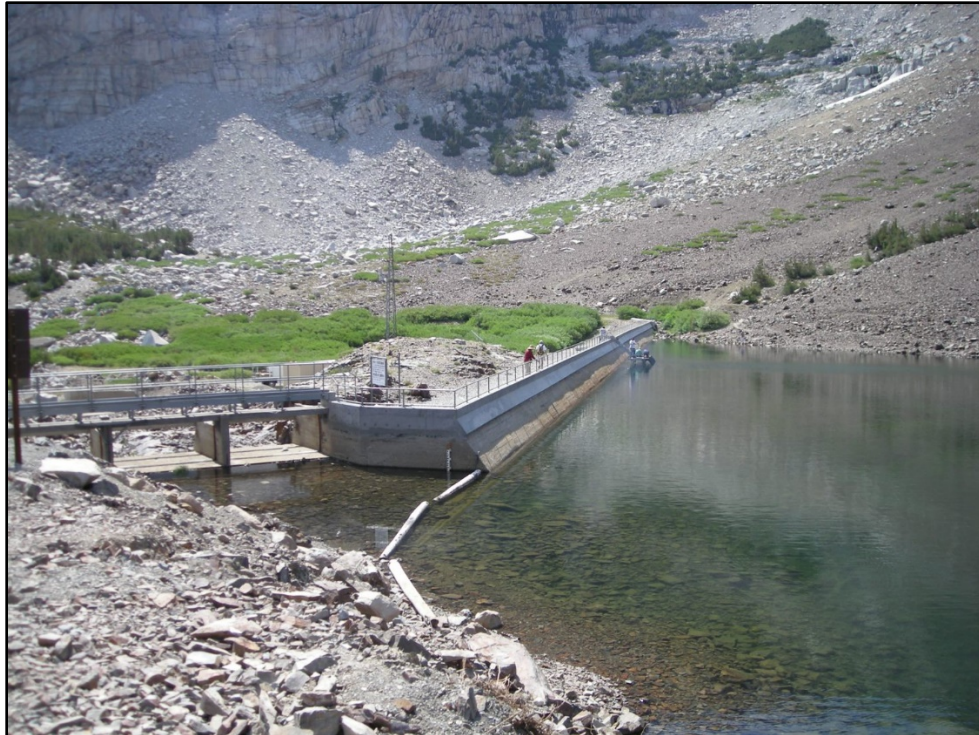
Photo 5.10-5. Rhinedollar Dam (Ellery Lake) and Spillway
