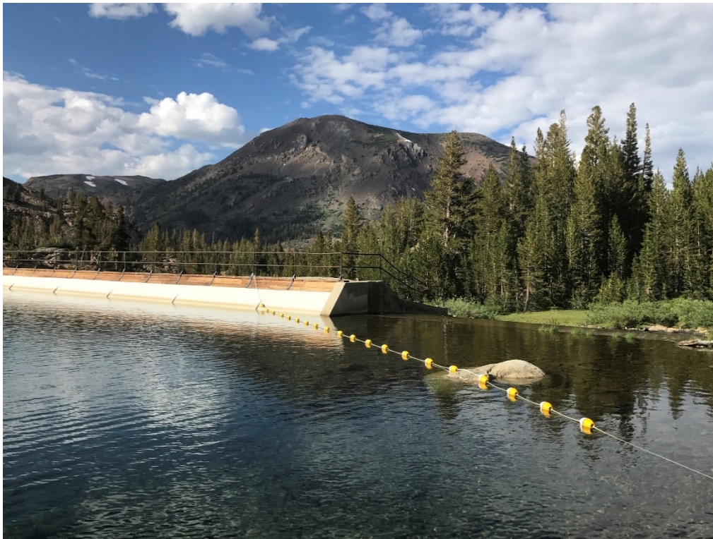
Photo 4.5-1. Tioga Dam and Spillway 2020
