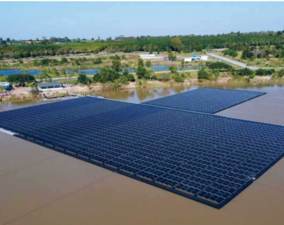
SCG Floating Solar Solutions in the Suranaree University of Technology's pond
