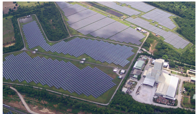
➤ Solar Farm at Kaeng Khoi Factory
