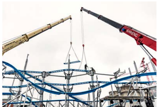
Ten trucks in total haul the roller coaster parts to the site: a huge jigsaw puzzle made of turns, cars and supports. Large boom cranes lift the components, some of which weigh several tons, into position. The whole installation takes three days
