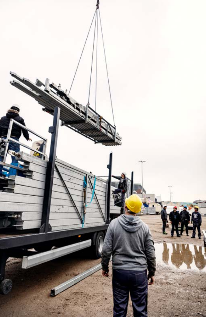
Ten trucks in total haul the roller coaster parts to the site: a huge jigsaw puzzle made of turns, cars and supports. Large boom cranes lift the components, some of which weigh several tons, into position. The whole installation takes three days
