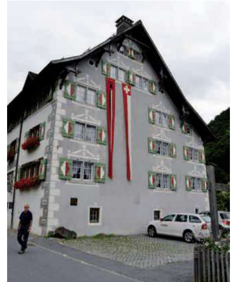
Suworow-Haus in Elm.
