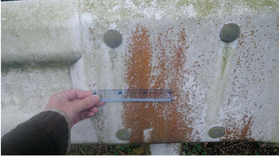
Figure 4. Terrestrial green algae growing on the surface of a highway guardrail. The cells form orange and dull green sections.
