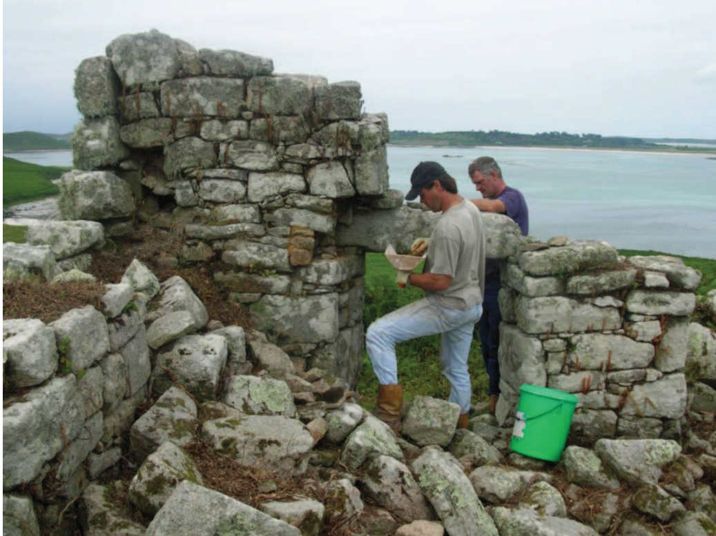
Fig 9.6 Consolidation work being carried out on House N on Samson in July 2006 (photo:Jacqui Mulville)
