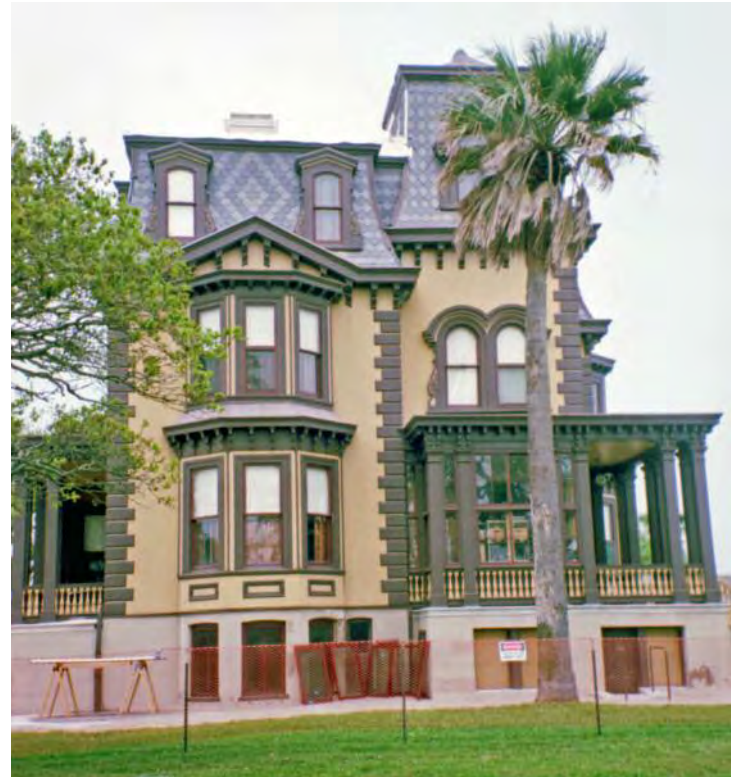
Aug. 2019: Repairs nearly complete on the Fulton Mansion. Original slate tiles from the damaged roof were collected, etched with inspirational words, and sold to help pay for repairs.
