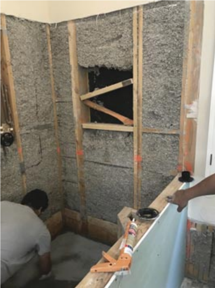
Bathroom in progress
