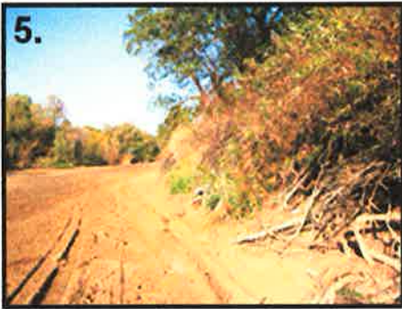
5. Out-of-place channel after fill and initial grading.
