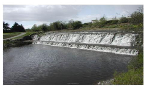
FIGURE 12: FIRHOUSE WEIR, THIS DIVERTED THE DODDER TO ENHANCE THE WATER SUPPLY TO 13<sup>TH</sup> CENTURY DUBLIN; RESEARCH HAS SHOWN THIS WEIR WAS CONSTRUCTED BY THE MONKS OF THE ABBEY OF ST THOMAS, THOMAS STREET, DUBLIN AND MODIFIED IN 1244 BY CITIZENS TO FURTHER ENHANCE SUPPLY (SDCC LIBRARY).
