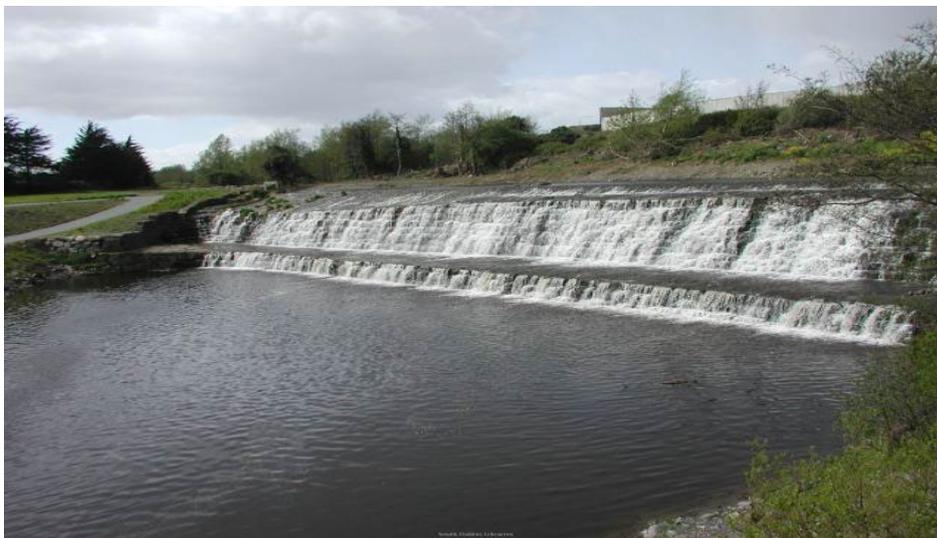
FIGURE 12: FIRHOUSE WEIR, THIS DIVERTED THE DODDER TO ENHANCE THE WATER SUPPLY TO 13<sup>TH</sup> CENTURY DUBLIN; RESEARCH HAS SHOWN THIS WEIR WAS CONSTRUCTED BY THE MONKS OF THE ABBEY OF ST THOMAS, THOMAS STREET, DUBLIN AND MODIFIED IN 1244 BY CITIZENS TO FURTHER ENHANCE SUPPLY (SDCC LIBRARY).
