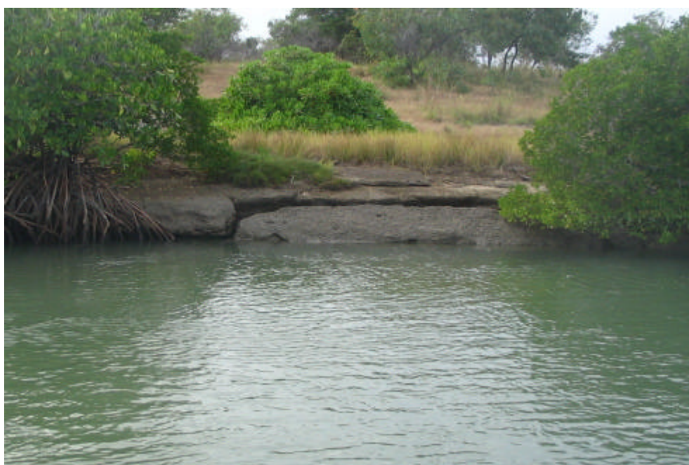
Figure 5.15: Undercut rock shelf along the shore of Triluck Creek, Albatross Bay.
