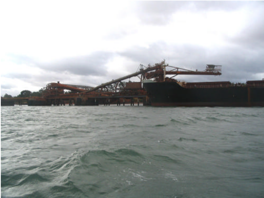
Figure 9.2: The bauxite ship loader at Lorim Point in the lower Embley estuary. This currently handles an average of 1 ship per day, limited by loading time and tides.
