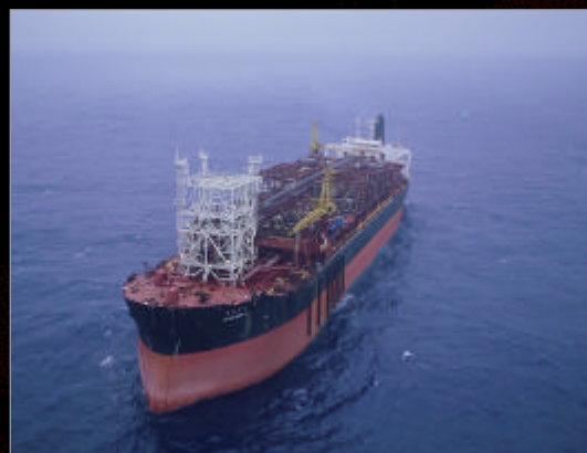
Floating Production Storage and Offloading/Turret Mooring System
