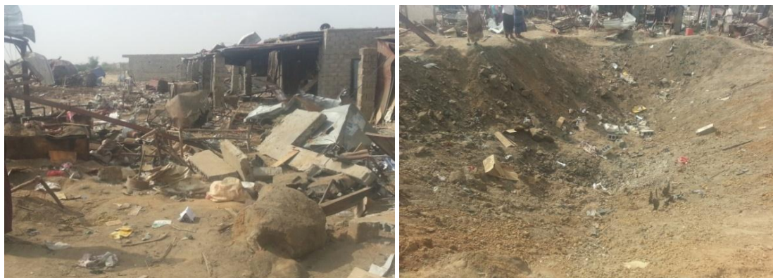
Figure II Damage to the Khamees market
