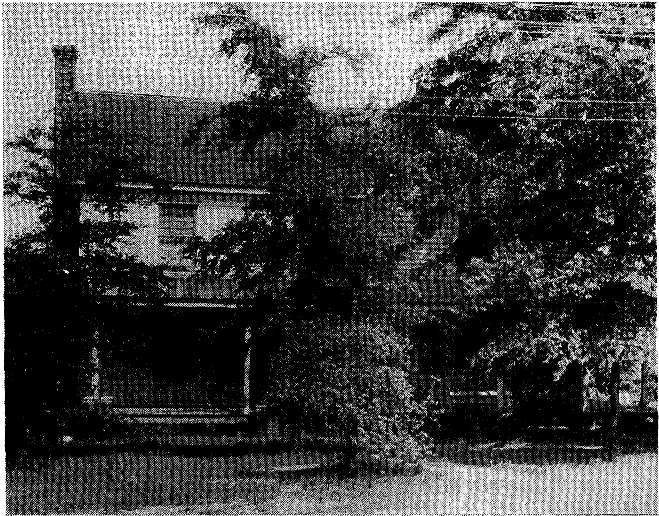
D. J. and Eliza Sanders home on Homer Street at the top of the hill. Built in 1872. Occupied by them until their death. An elevated point in the city.
