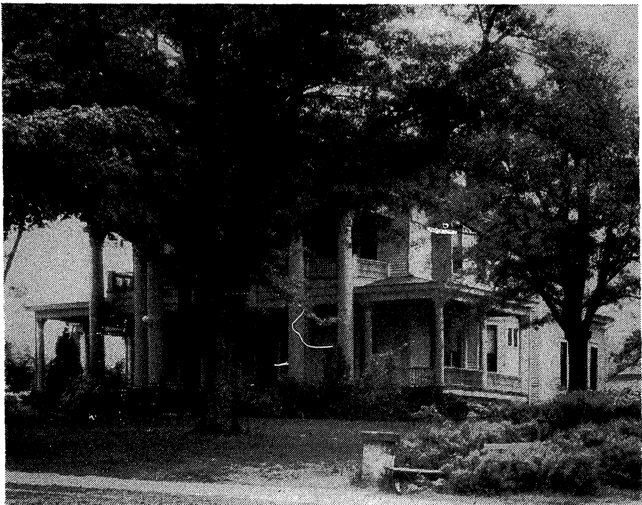
Photograph of the same building as above in 1948. 114 South Elm Street.
