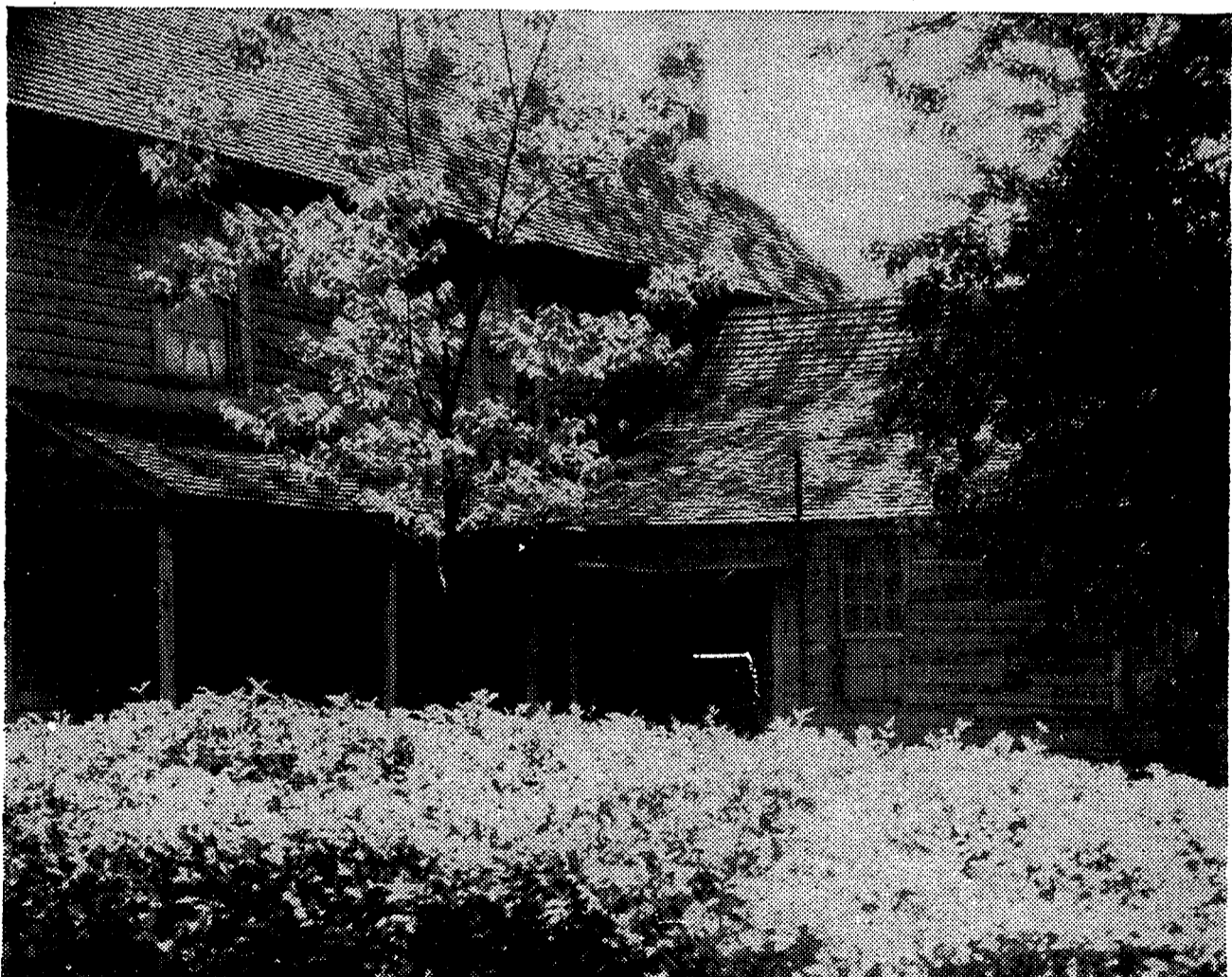
Rear view of the Northeastern Hotel showing the kitchen and back veranda.
