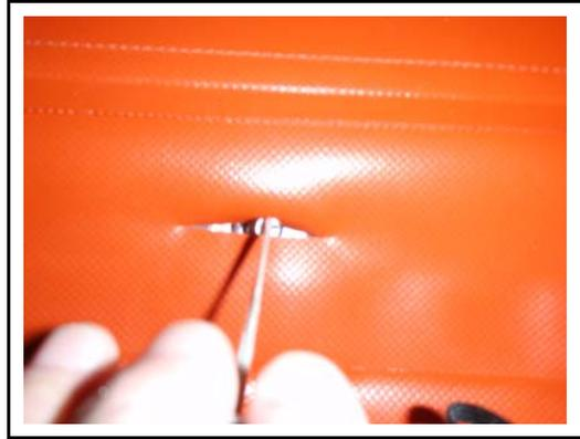
4. Place the top of the clamp over the bolt.
