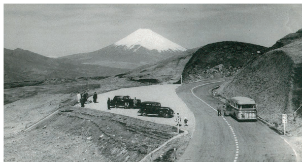
Expressway built by Sunzu Railway
