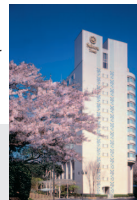
Takanawa Prince Hotel Sakura Tower
