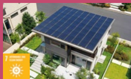
A large capacity solar power generation system
