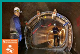
Sewage (Spirally) Pipe Renewal (SPR) Method
