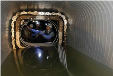
"SPR Method," with the advantage of "No-dig installation"
