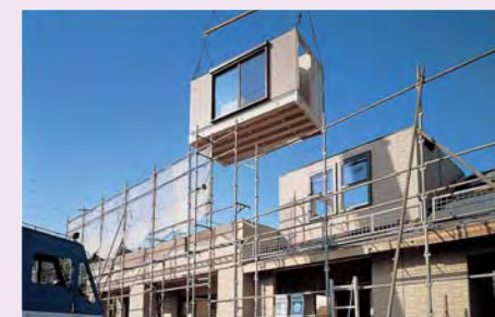
Swift on-site assembly completed in just one day
