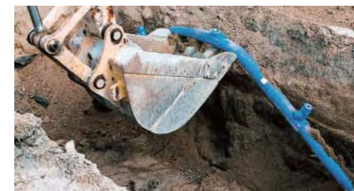
Esilon Hyper JW (polyethylene pipe), capable of resisting earthquakes
