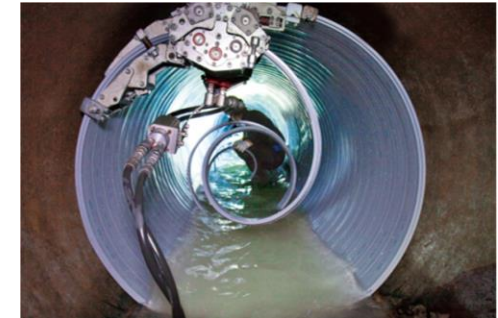
Sewage (Spirally) pipe renewal (SPR) Method
