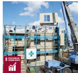
A housing unit being installed
