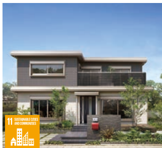
External walls ( Eco-chante ) renovation
