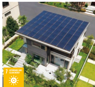
A large-capacity solar power generation system
