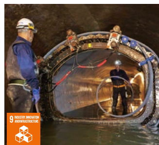
9 INDUSTRY, INNOVATION AND INFRASTRUCTURE Sewage pipe rehabilitation
