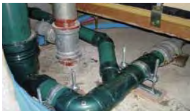
Seismic and fire-resistant retrofitting and construction stock-related demand is growing in the domestic core businesses (Photo: ESLON fire-resistant VP pipes).
