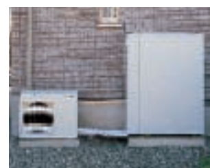
Hot Water Unit with CO 2 Heat Pump
