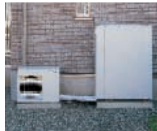
Hot Water Unit with CO 2 Heat Pump
