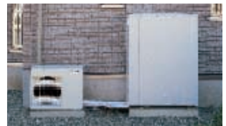
Hot Water Unit with CO2 Heat Pump
