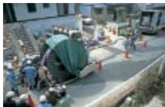
▲Work in a built-up residential area
