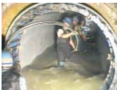
▲Relining of a sewer pipe while effluent flows
