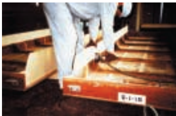
Reinforcement work of a water treatment tank cover after use for about 20 years
