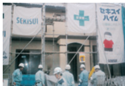
A safety check is performed at a construction site.
