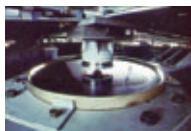
Seismically isolated bearing
