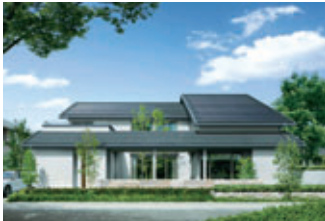
IS ORDER steel-frame detached house
