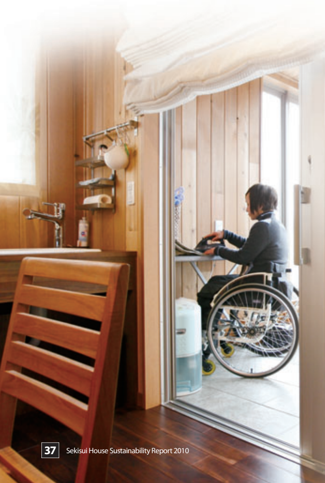
An in-door sunroom constructed in place of the deck includes a floor flush with the house, allowing for easy wheelchair access.
