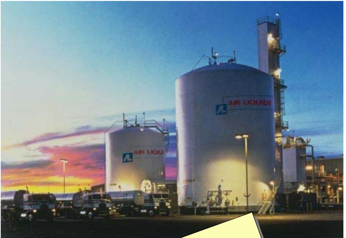
Photo: Air Liquide
