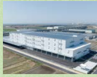
Installing solar power and energy-saving equipment at PD centers
