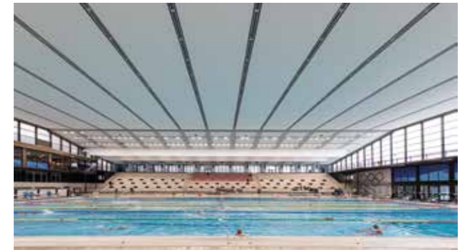
Olympic swimming pool, Naples ■ Italy
