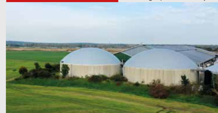
Biogas plant ■ Germany
