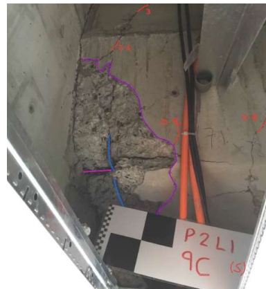
Pier 2, Grid C/9 Level 2 beam
