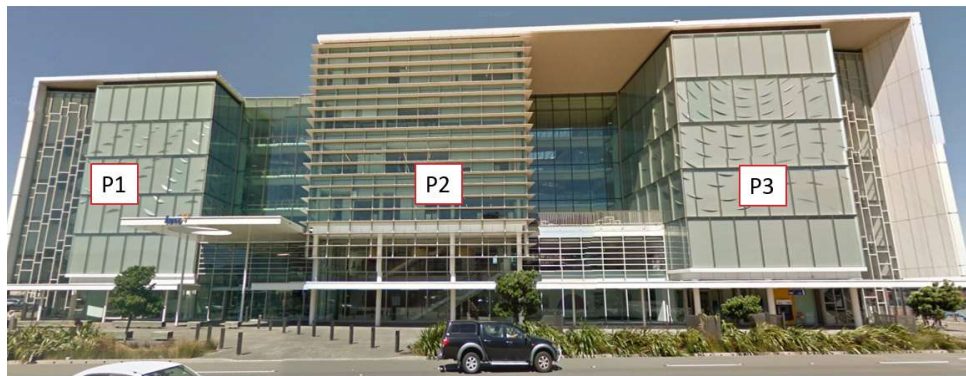
X Axis (along the Link Bridges) North South
