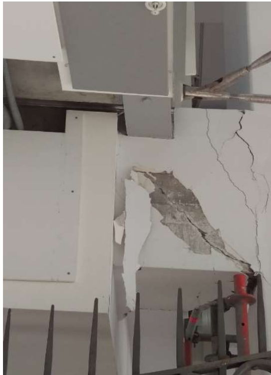
Pier 2 L1 Grids 6 and V beam
