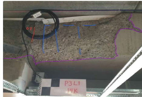
Pier 3, Grid 14/K Level 2 beam
