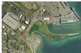
Aerial View. Source: Bing Maps
