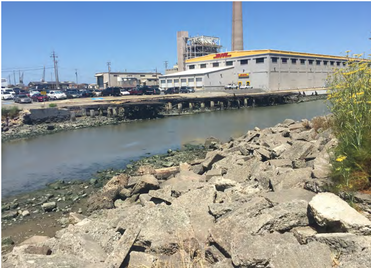
Representation of riprap to stabilize shoreline
