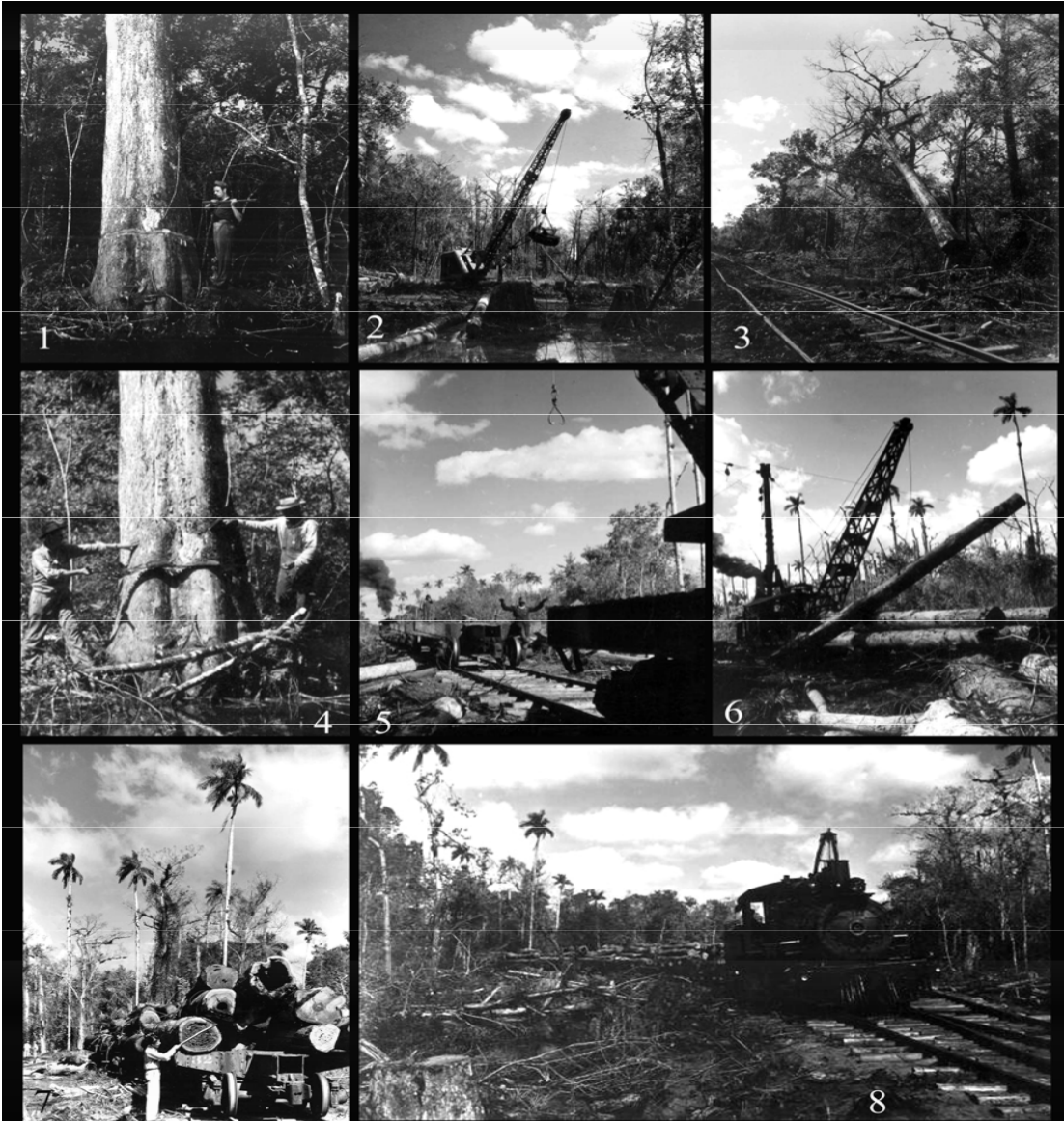
Figure 5. Tram Logging: 1) scouting parties girdle virgin cypress up to a year before logging to allow the stored water to drain out; 2) tram roads are created with a diesel dragline that dredges adjacent soil and muck to build up the road bed; 3) narrow gauge rails are laid on the tram roads, called "dummylines"; 4) logging teams fell the trees; 5) rail cars forming a train; 6) steam skidder loading cypress logs; 7) measuring the diameter of felled logs; and 8) hauling the trees to a local mill which, at its peak, was producing 100,000 board feet of lumber a day.
