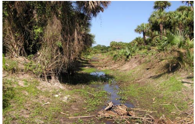
Toney Strand Project before sediment removal.
