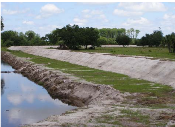
Perimeter berm being constructed around Retention area.
