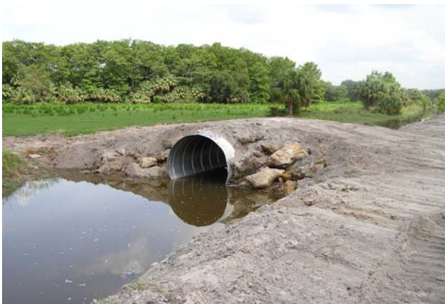
A cattle crossing installed on the Toney Strand. The crossing reduces cattle access within the waterway.
