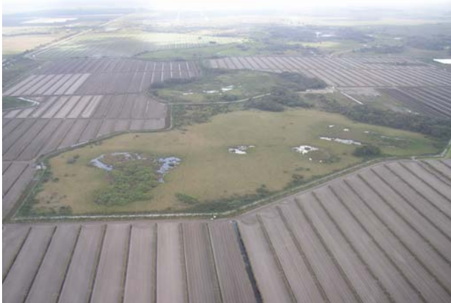
The picture above is an aerial overview depicting a portion of the J-7 Ranch Project's row crop operation before construction. The green area will serve as the D-1 and D-2 detention areas.
