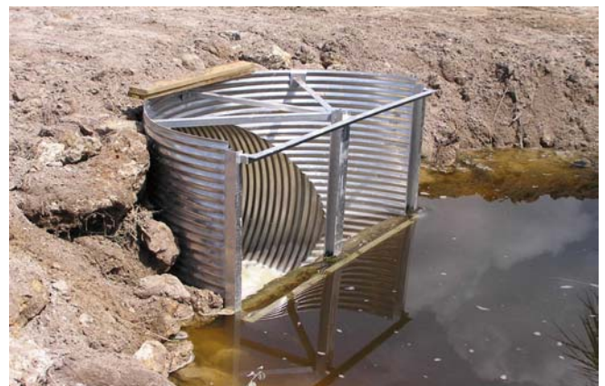
Culvert with header and sediment boards installed as part of project.
